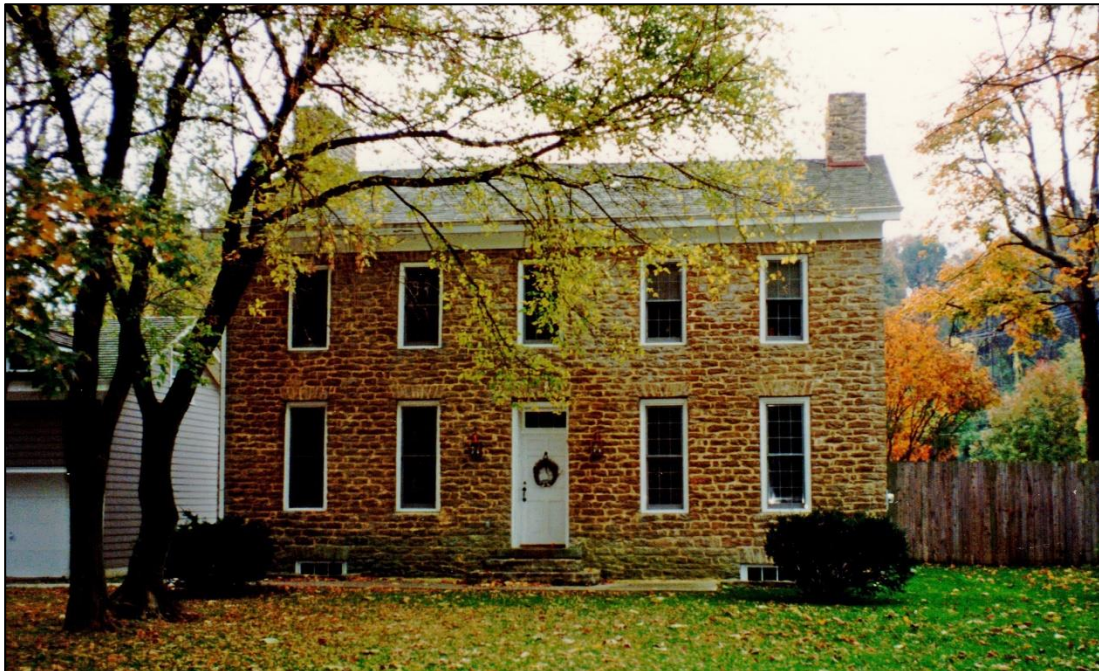
Elliott House after the renovations, which started in 1985
