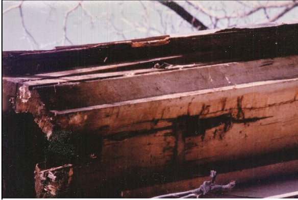
Portion of log gutter found during restoration
